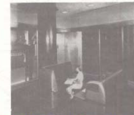
The IBM SSEC-Selective Sequence Electronic Calculator (Circa 1950) Designed by John VonNeumann in 1948, the SSEC, built by IBM, operated through the use of 13,000 vacuum tubes, some of which can be seen against the back wall (left in this photo). Courtesy of IBM - International Business Machines
